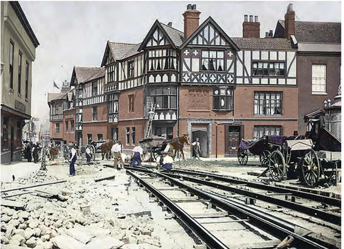
Tracks are laid from Tombland along Wensum Street in front of the reconfigured Maids Head, c.1899
